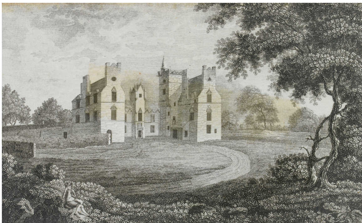
Wrytes Houses adjacent to Bruntsfield Links, by A. Robertson
